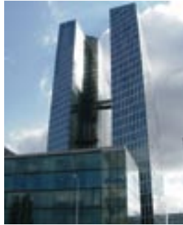
Figure 3 – Highlight Towers – Munich (under construction)
